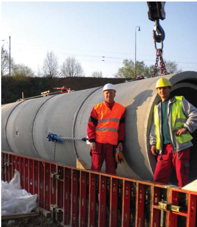
D3 Votice Construction of D3 culvert – side installation DEHA Pipes TZh DN 1600
