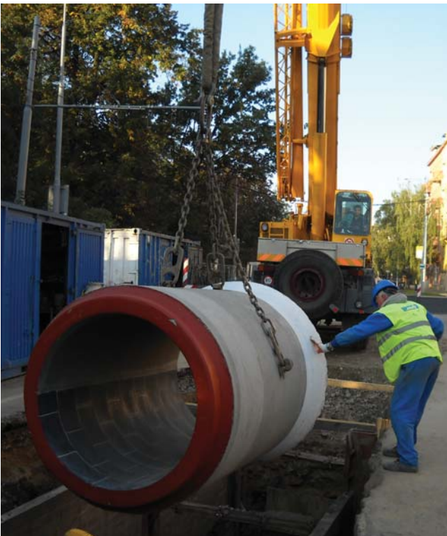
Brno – Pionýrská Street – Reconstruction of sewer network - TZh DN 1200 CV 180
