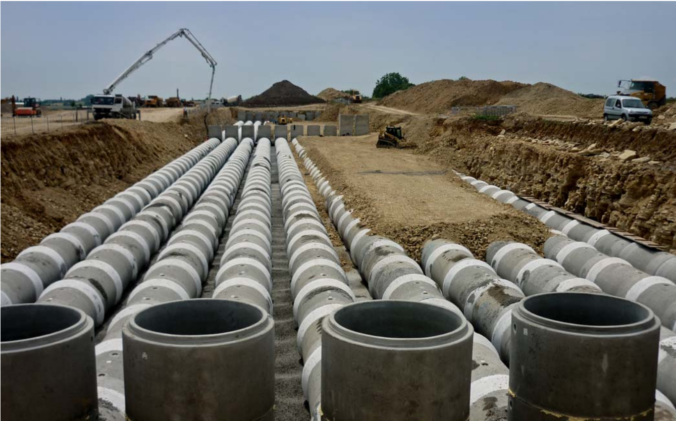
LEGO KLADNO – Construction of retences in Kladno industrial zone - TZh DN 1200
